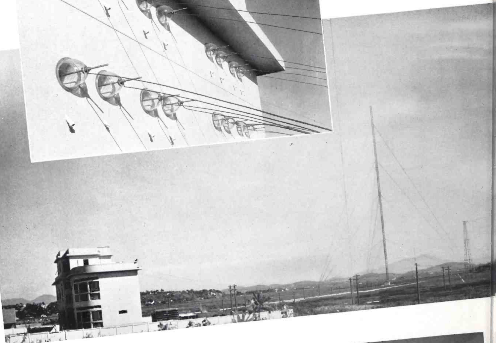
WAR WEAPONS IN LAND OF CARNIVAL —Panoramic view of the group of Radio Nacional's eight antennas rising against majestic backdrop of Brazil's mountains. Five of these antennas are directional and three non-directional. Two directional antennas (16 and 25 meters) are beamed to the United States, two others (16 and 25 meters) to Europe, and a fifth (25 meters) to Asia; while the remaining three non-directional antennas operate on the 16, 25 and 31 meter bands. This group is suspended on six 105' galvanized steel towers.
