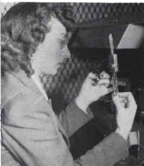
The completed rebuilt filament stem with new filament installed.
