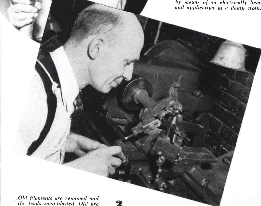
Rebuilt anode with new, thick copper cone ready for machining to obtain new feather-edge for glass-to-metal seal.
